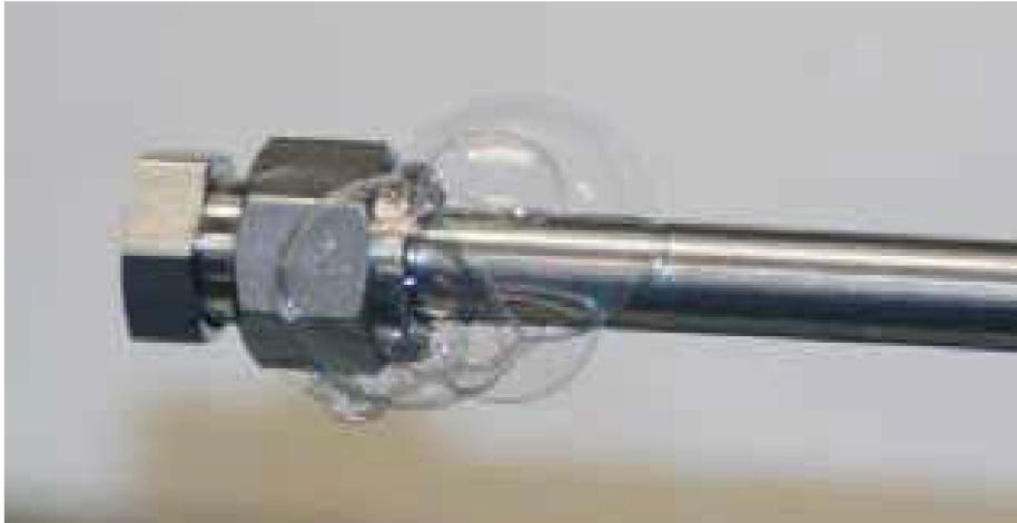
Figure 10-8 Larger leak displays large bubbles.
