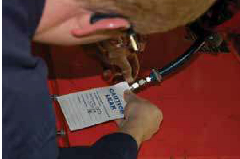
Figure 10-11 Detect and identify leaks.
